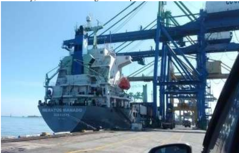
Figure 2. Quay Container Crane (QCC)
