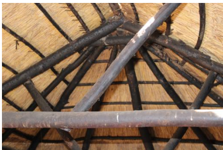
Fig. 5: Roof strengthening technique in Ndebele Hut
